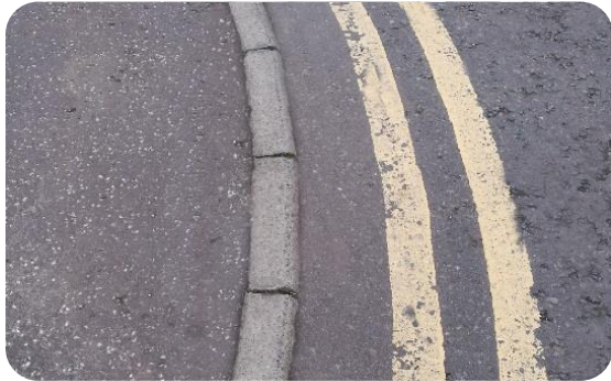
Grade A (compliance) Road is free from detritus
