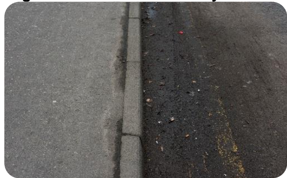
Grade D Road surfaces are obscured or at high risk of hazard caused by detritus
